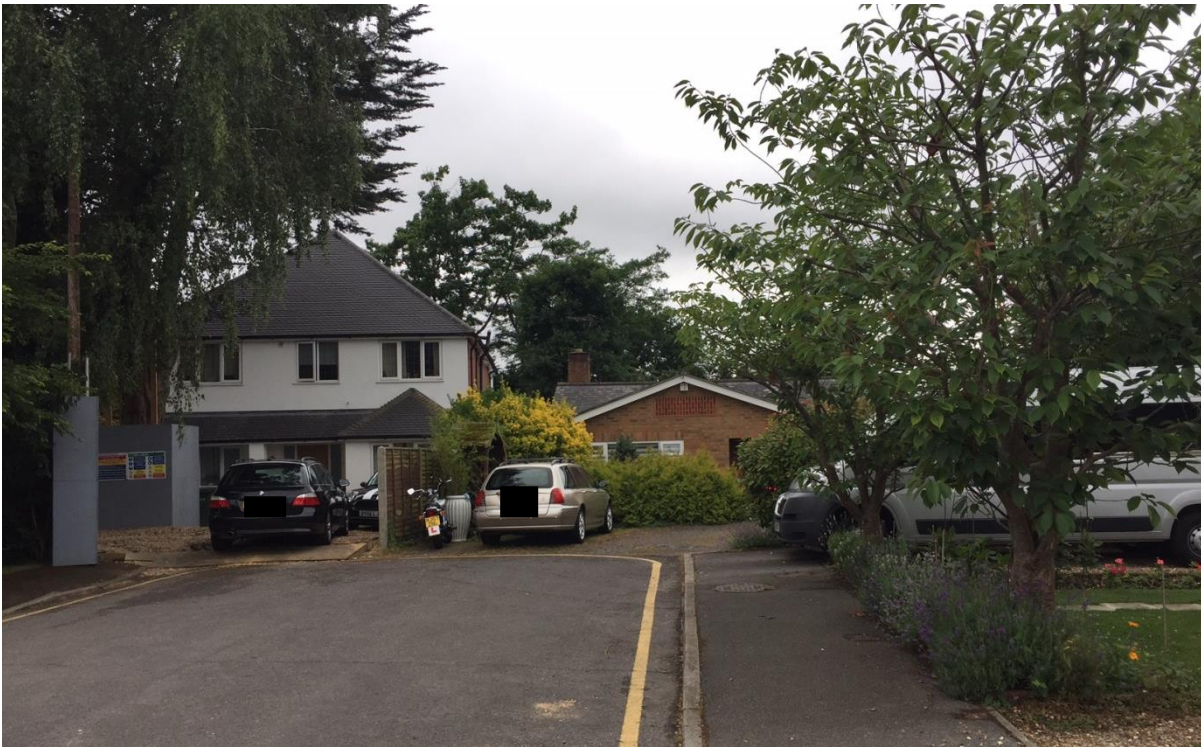
Existing front elevation of the subject property.
